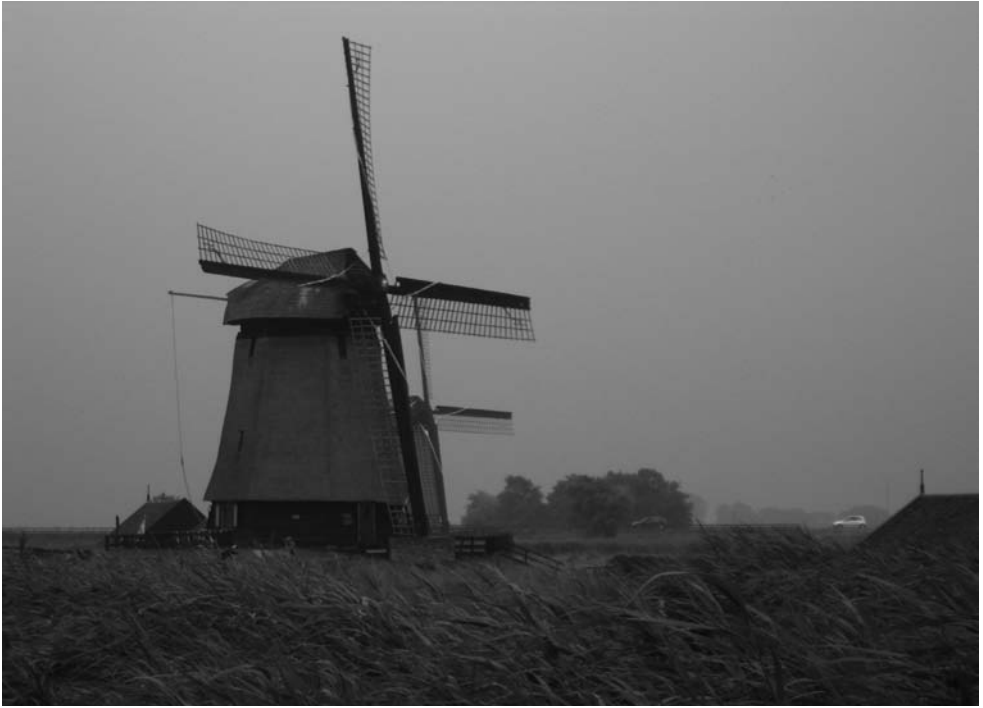
Figure 6.2 Drainage windmills in the Schermermeer polder, Netherlands. These provided energy for machines such as the Archimedes screw pump to raise water into canals and make land available for agriculture. Photograph taken in 2007.
