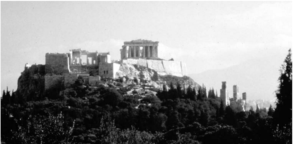
Figure 4.1 The Parthenon and other buildings in Athens, Greece, crown the Acropolis, a limestone outcropping around which the city grew. The stone used in their construction is marble brought from Mount Pentelicus, 13 km (8 mi) distant. Photograph taken in 1966.
