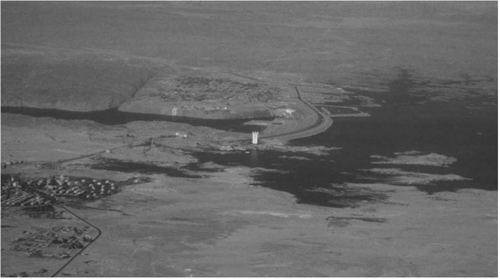
Figure 7.5 Aerial view of the Aswan High Dam on the Nile River in Egypt; Lake Nasser to the right. This dam, which ended the annual flooding of the Nile below it, impounds two years' flow of the river. It has been hailed as one of the greatest projects of the twentieth century and denounced as a major ecological catastrophe. Photograph taken in 1981.
